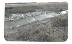
In order to address the head cutting occurring downstream of the concrete drop structures installed in the 1950's by the US Army Corps of Engineers, the Sand Hill River Watershed District worked collaboratively with the Minnesota DNR, the Board of Water and Soil Resources, and the West
